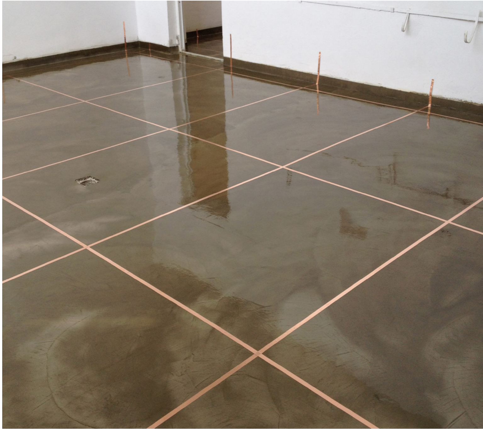
ELECTRONICS AND ELECTRICAL ENGINEERING Antistatic/conductive epoxy covering specifically for IEC 61340 areas made with NORPHEN ESC.
