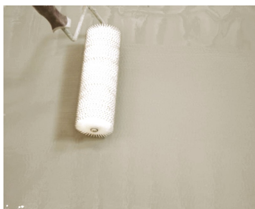
Figure 4 - Use of the spiked roller for the second coat.
