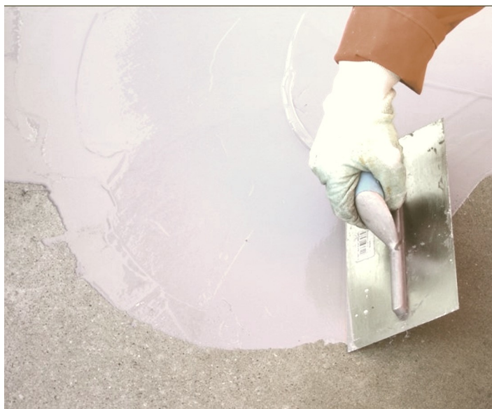
Figure 2 - Skim coating on concrete.
